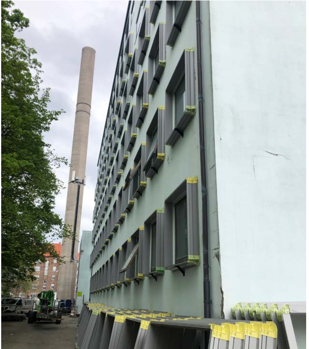
The corner profiles, which can be green, yellow, or brown, are manufactured from recycled plastic sourced from the dairy industry.
