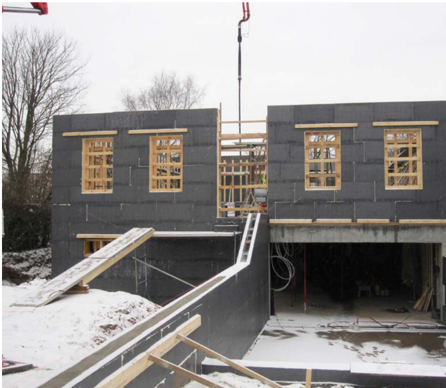
The element in use in the building process.
