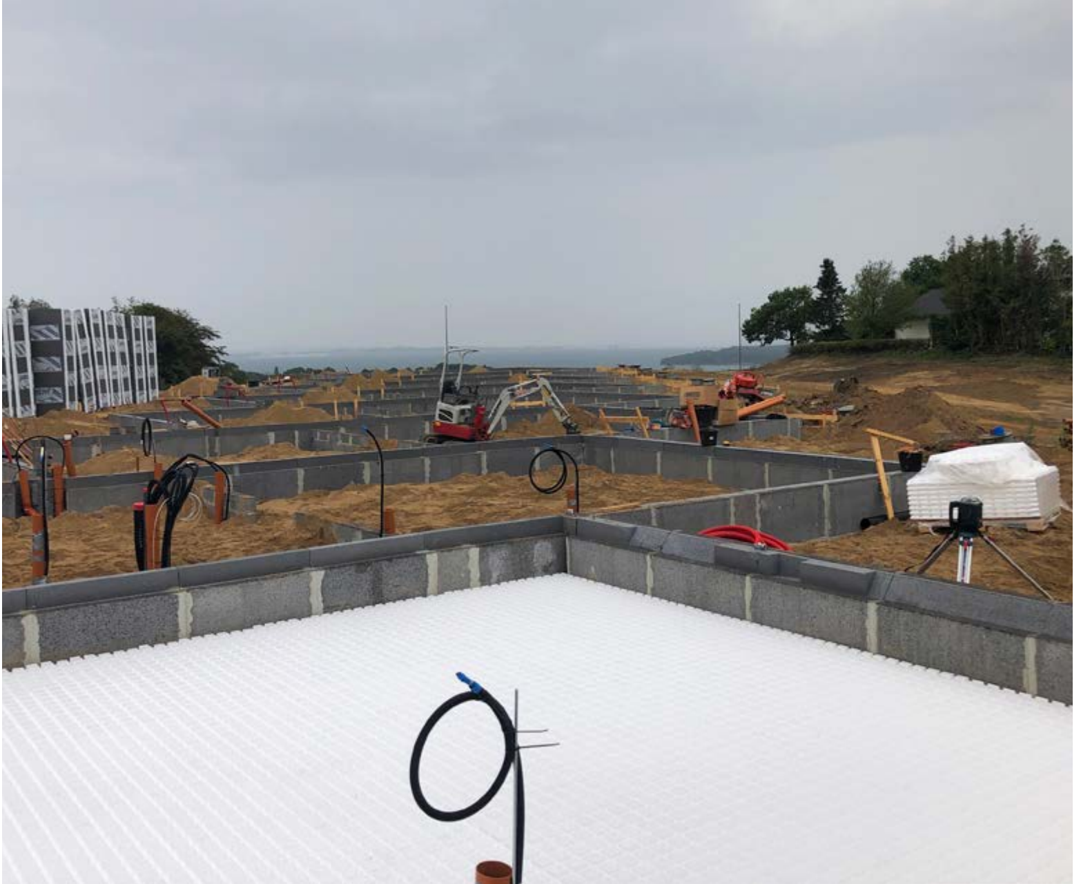
Contractor Møllerens Hus A/S used the plates in the construction of 29 houses in Ugelbølle, Mols, Denmark, to protect the buildings against radon in the soil.
