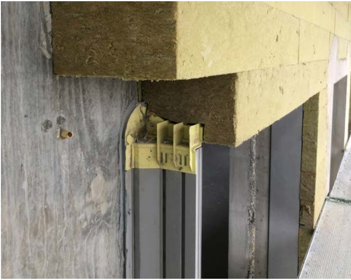
The corner profiles, which can be green, yellow, or brown, are manufactured from recycled plastic sourced from the dairy industry.
