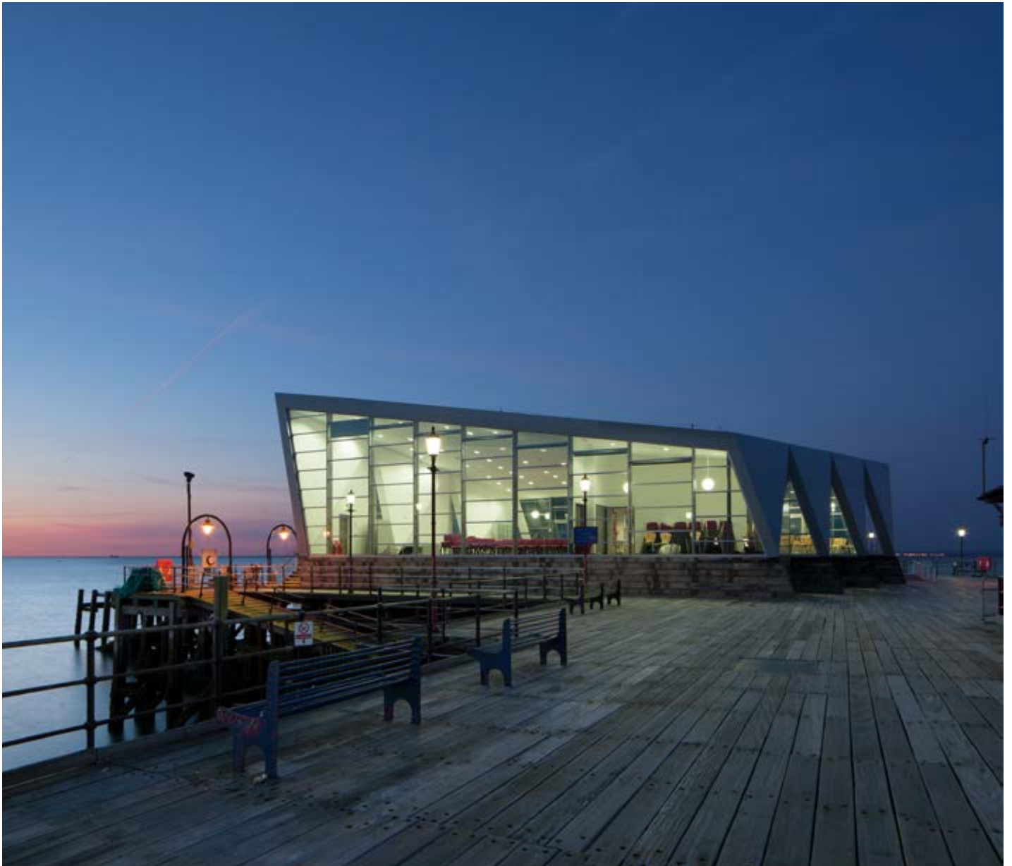
Fibreglass facade planks used for the Cultural Center on Southend Pier, Essex. Architects: White Arkitekter & Sprunt.
