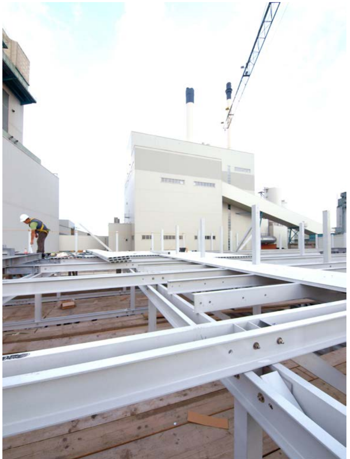
Bridge made with fibreglass profiles.
