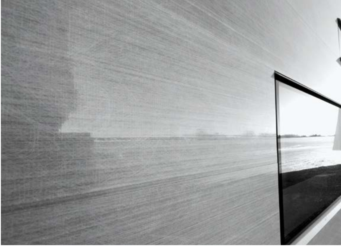
Close-up of fibreglass facade planks.
