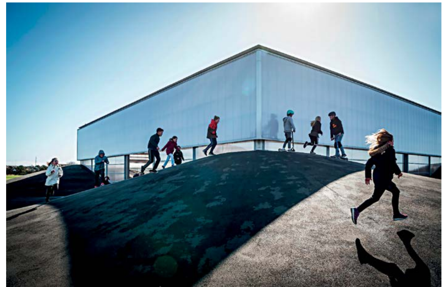
The panels were used in the Harboore Activity Center in Western Jutland by JAJA Architects in 2015.
