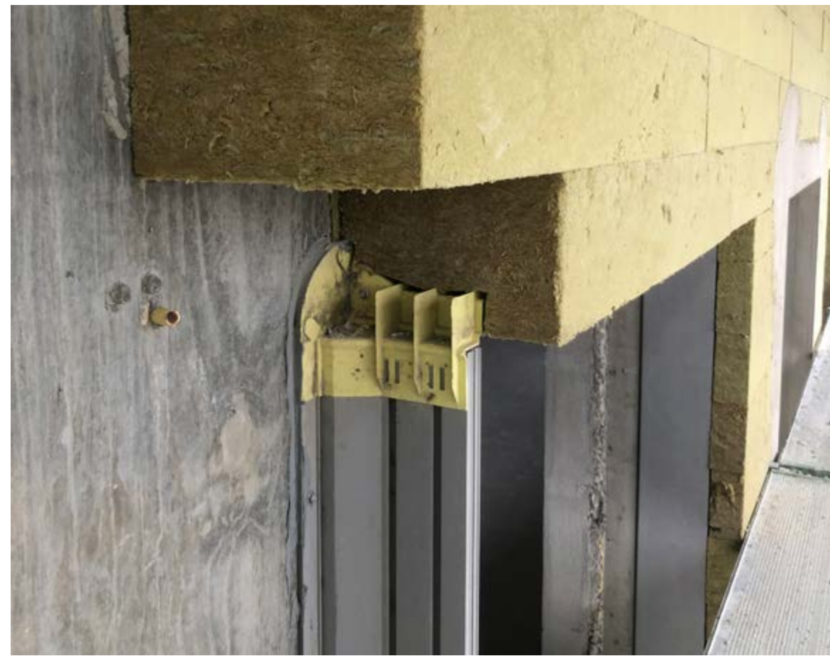
The corner profiles, which can be green, yellow, or brown, are manufactured from recycled plastic sourced from the dairy industry.
