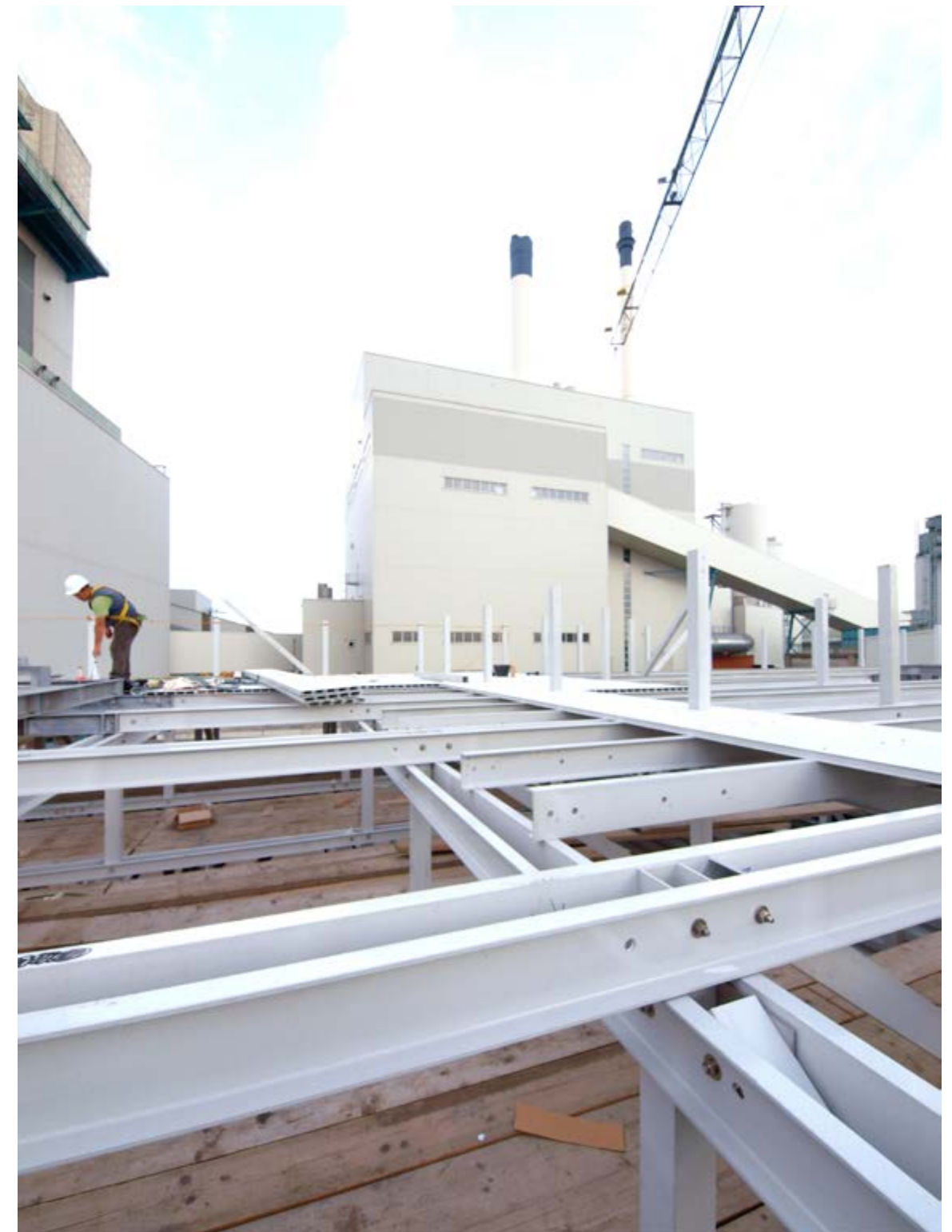
Bridge made with fibreglass profiles.
