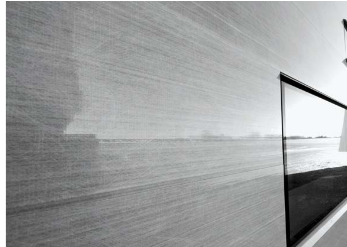
Close-up of fibreglass facade planks.
