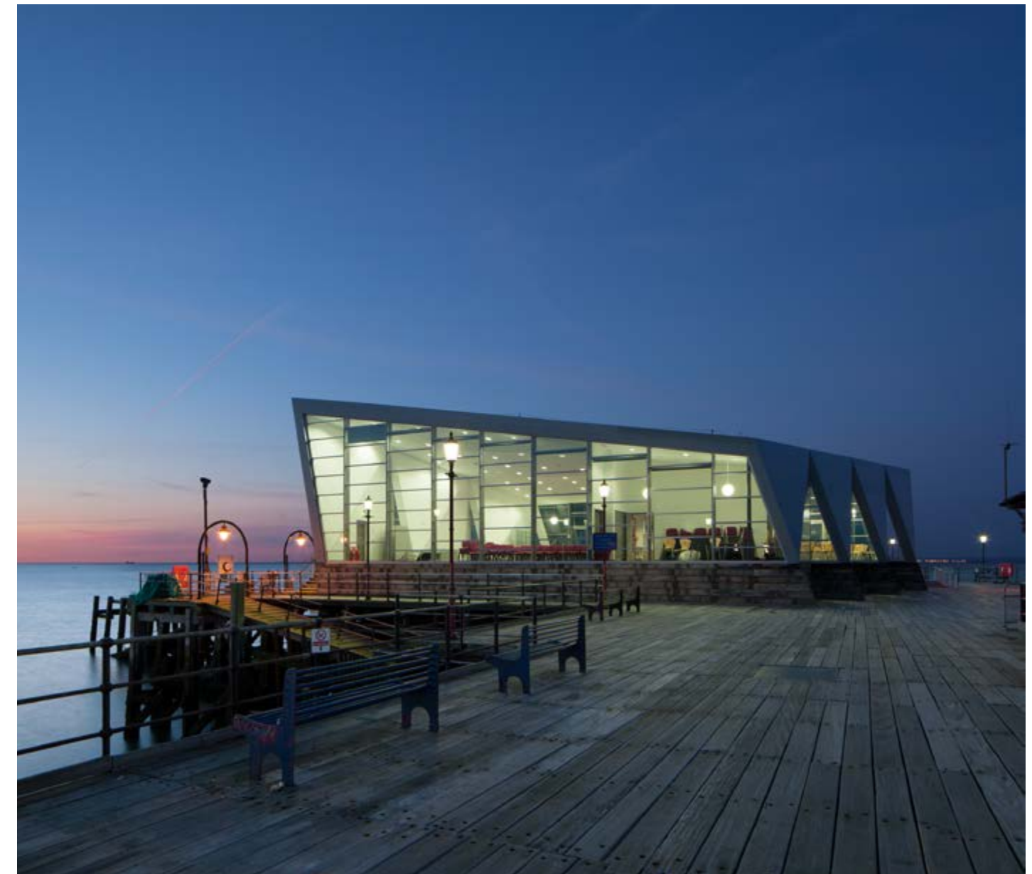
Fibreglass facade planks used for the Cultural Center on Southend Pier, Essex. Architects: White Arkitekter & Sprunt. Photo: Luke Hayes
