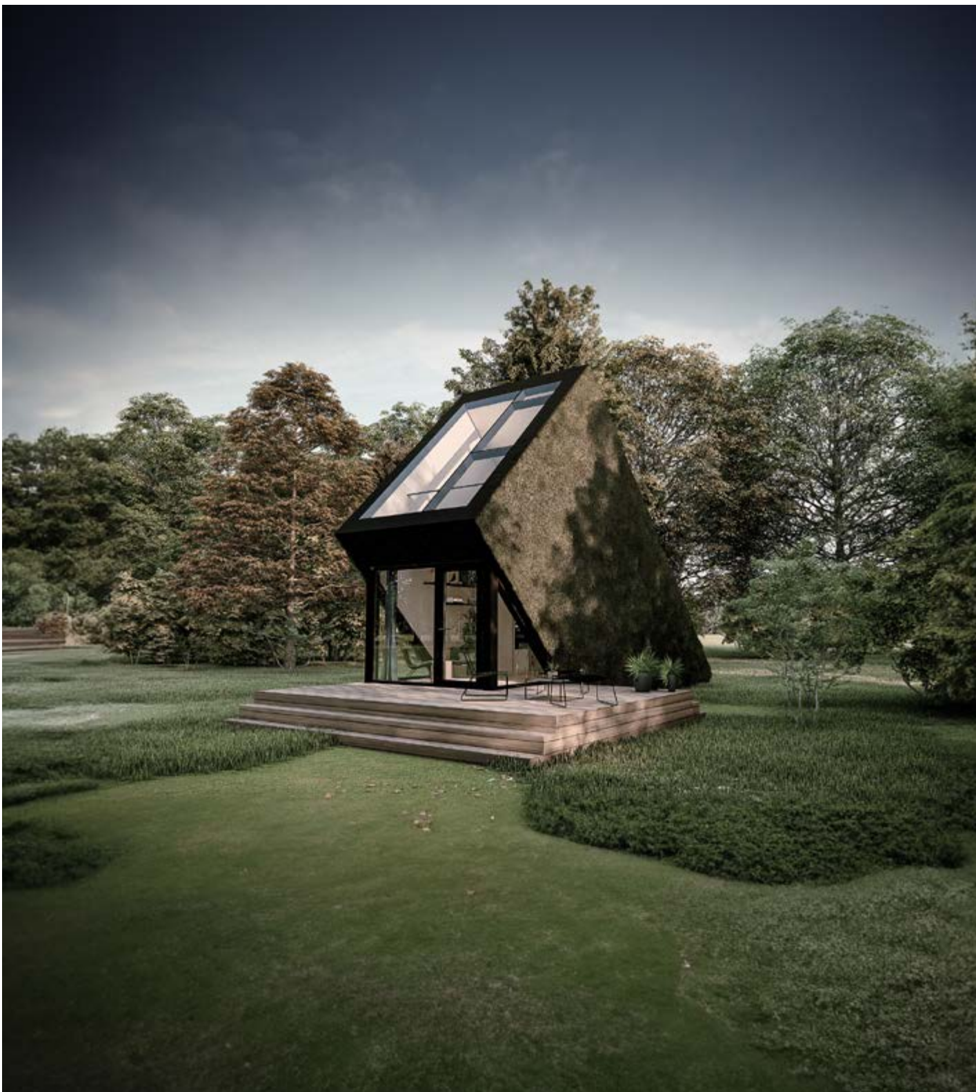
QUBEzero – a tiny house constructed using Smart Panels.
