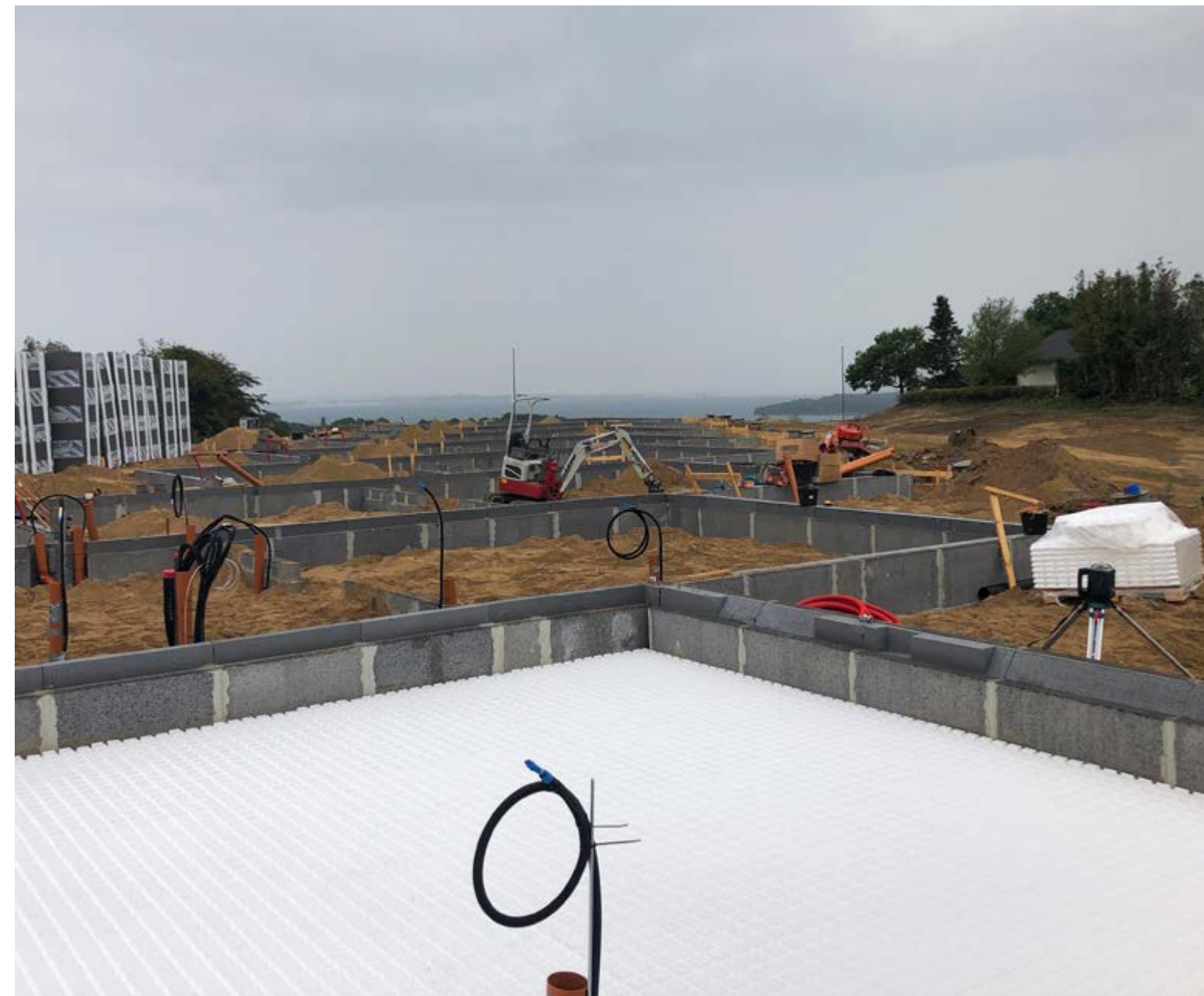
Contractor Møllerens Hus A/S used the plates in the construction of 29 houses in Ugelbølle, Mols, Denmark, to protect the buildings against radon in the soil.
