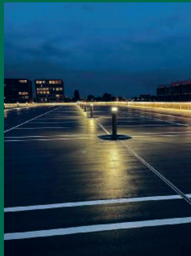
Example: Fiberline's car park system – lightweight temporary constructions that can be taken apart and used again in many places.
